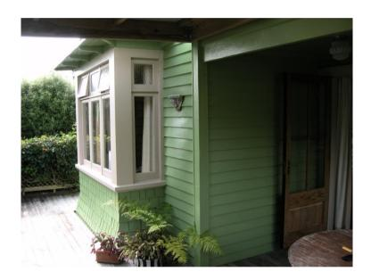
The House inspected is of a conventional timber construction with timber weather board cladding, wooden joinery and corrugated iron roof.
